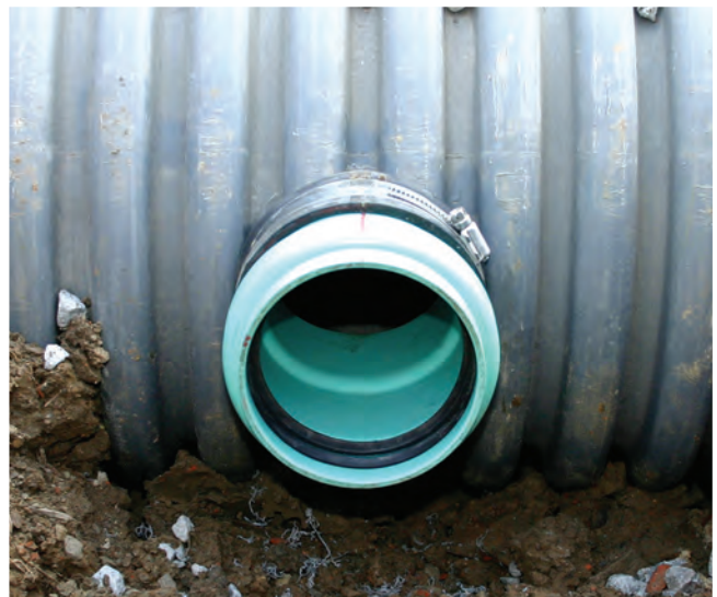
Inserta Tee Lateral Connection
